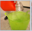
2. To a clean mixing bucket, add 6.5-7 litres of clean water depending on preferred consistency.
